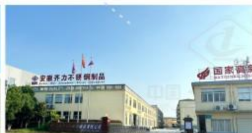
齐力集团安徽工厂 Qili Group Anhui Factory
